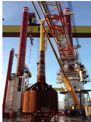
Fig. 1 Large-scale monopod bucket foundation on the deck of a jackup vessel (courtesy of Universal Foundation A/S)
